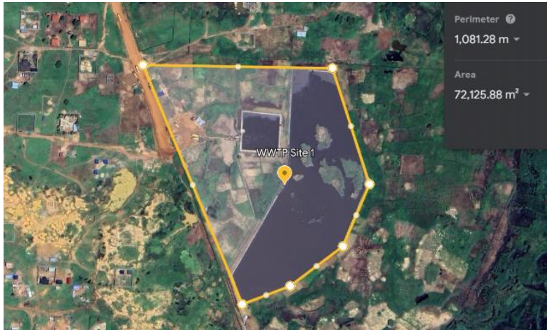
Figure 1: Existing Faecal Sludge treatment plant at Rokwe (Roton)
