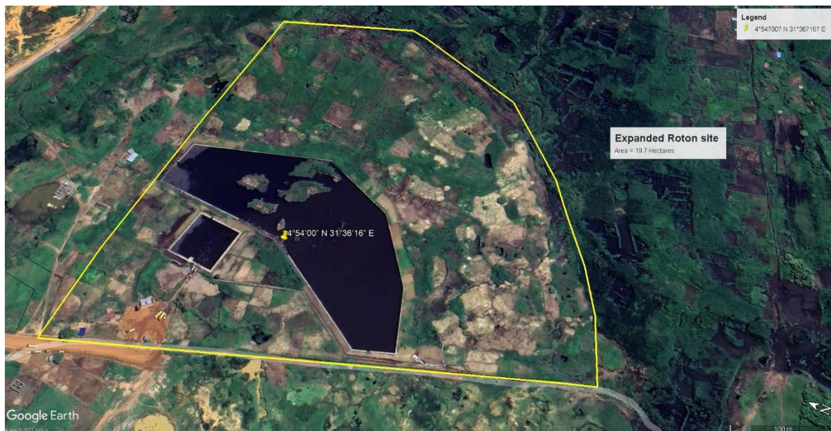
Figure 4: Project map (the full designated site of the wastewater treatment facility at Rokwe)
