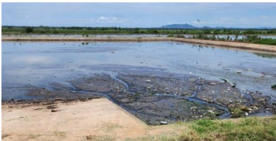
Figure 2: Existing Anaerobic Pond at Rokwe (Roton)
