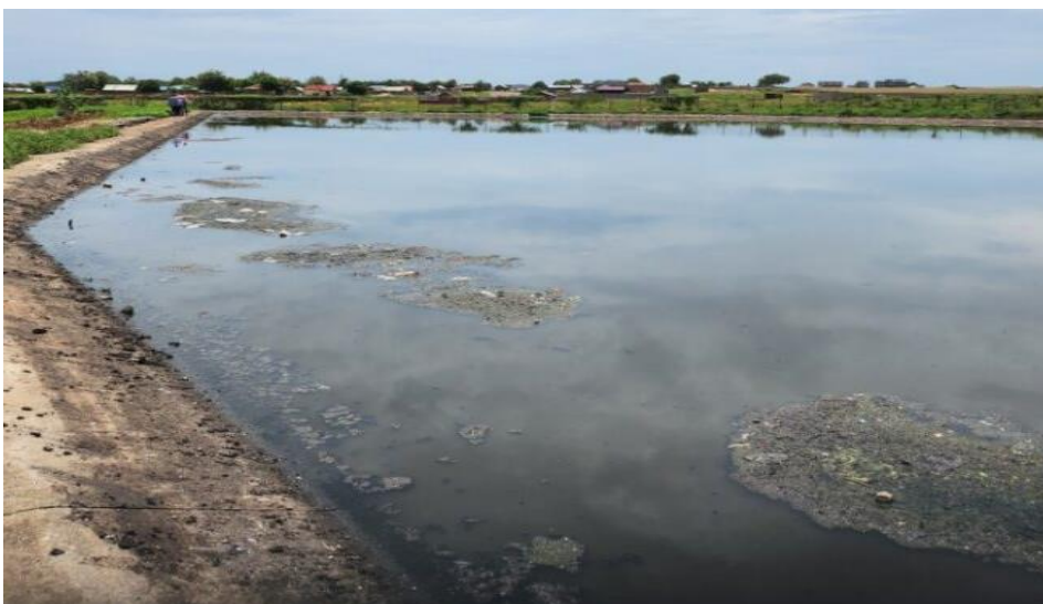
Figure 4: Existing Facultative Pond at Rokwe (Roton)
