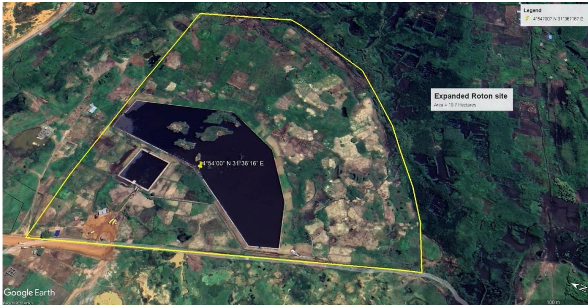
Figure 19: The location of the suitable site is enclosed in a yellow polygon
