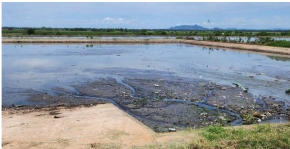
Figure 3: Existing Anaerobic Pond at Rokwe (Roton)
